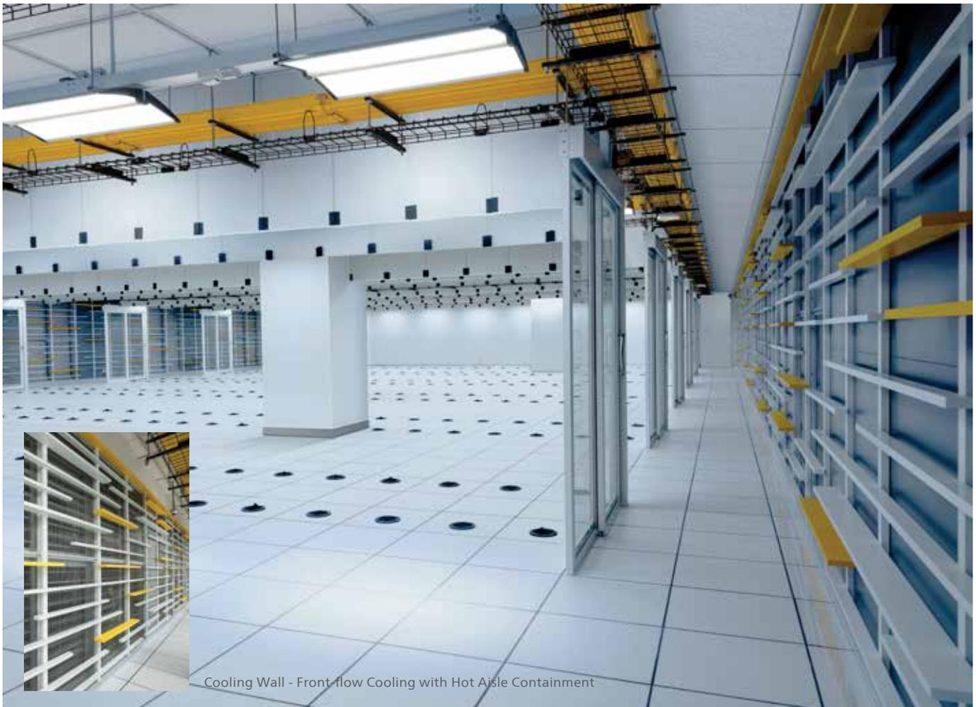
Cooling Wall - Front-flow Cooling with Hot Aisle Containment
